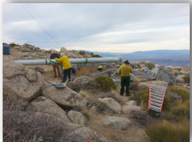
Tower pieces were picked and placed using a portable tripod rigging system.
